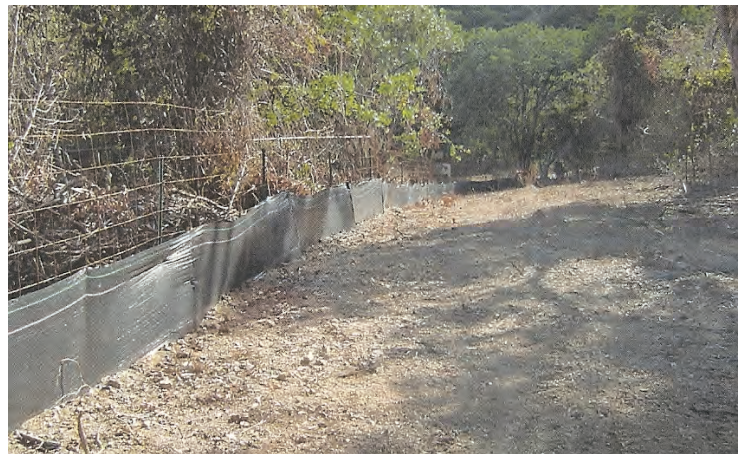
Silt fencing-used to prevent soil from leaving area and entering waterways.
